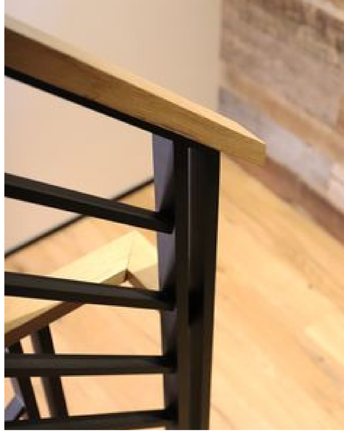
Metal Railing With wood stairs and Handrail
